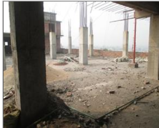
External photo(s) of the production unit(s) Construction work is going on.JPG
